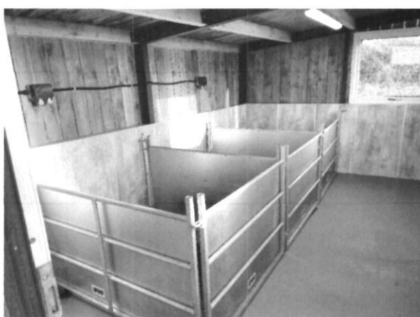
Our new quarantine building and pool.
