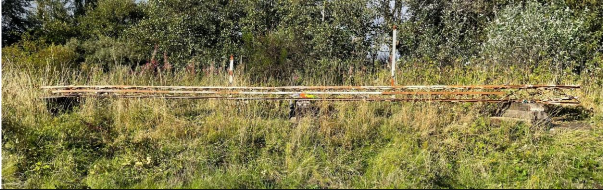
The TrAcS signal at Bo'ness undergoing paint removal and metalwork assessment
