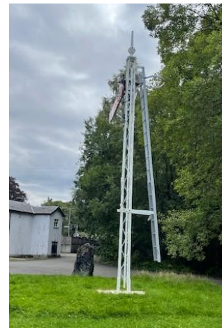
The signal near Pitlochry Station, showing the shortened ladder. David Ferguson
