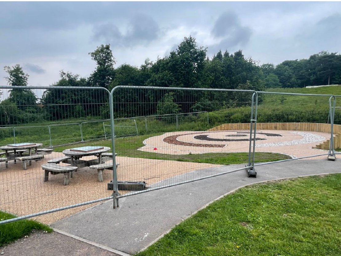
Sensory Garden during construction
