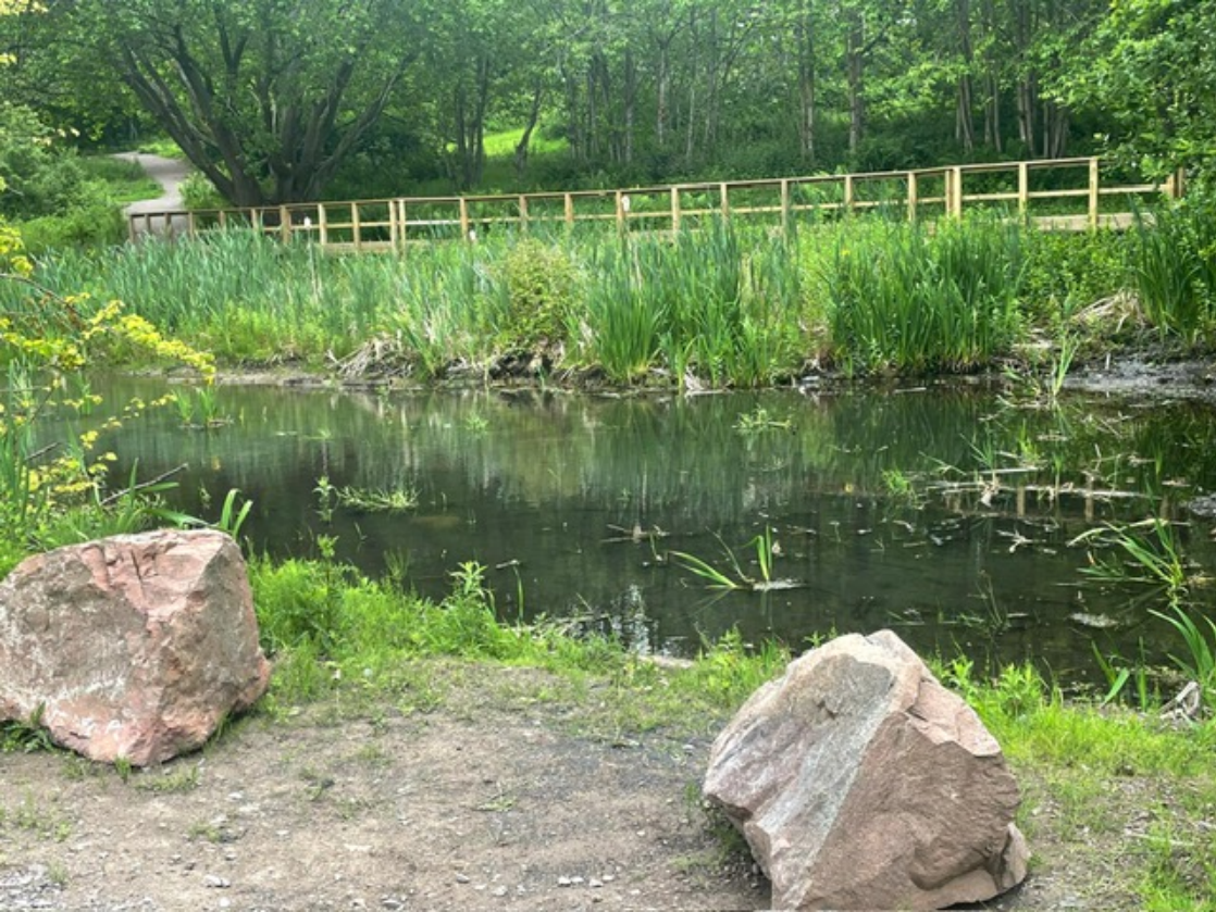
Boardwalk over Wetland Area during construction
