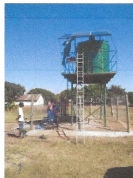
Secured Borehole site
