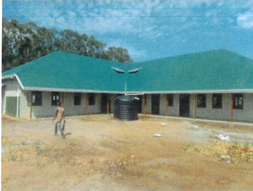
Boys Dormitory nearing completion
