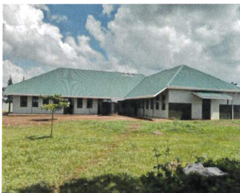
Completed Girls Dormitory
