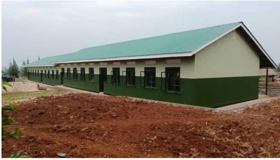
New 4 classroom block
