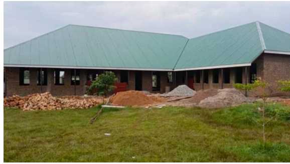
New Girls Dormitory being built
