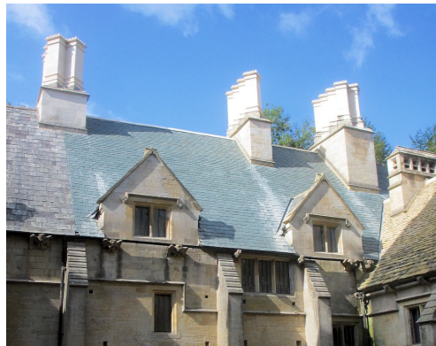
The new green slate roof on the N range, with restored chimney stacks, and to the right, the new Cotswold slate roof on the ironing room
