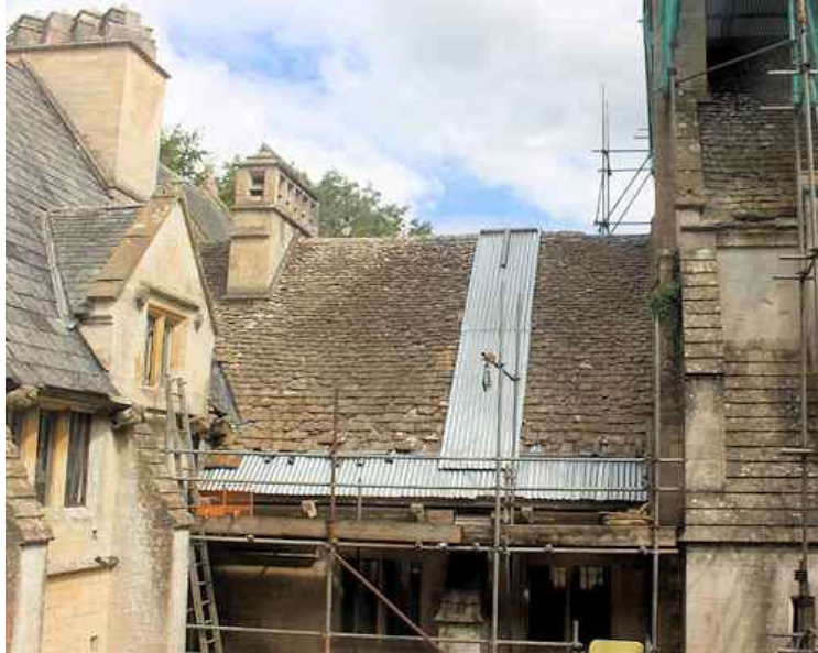
Ironing room roof before repair, showing corrugated iron patching, and to left, north range roof and chimneys awaiting restoration
