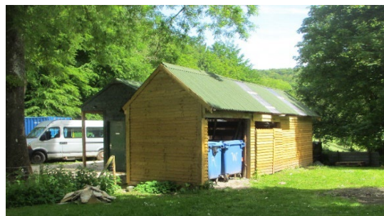
Shelter for rubbish bins and lawn mower constructed by maintenance volunteers.
