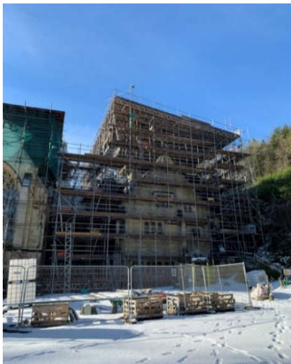
Scaffolding and overroof
