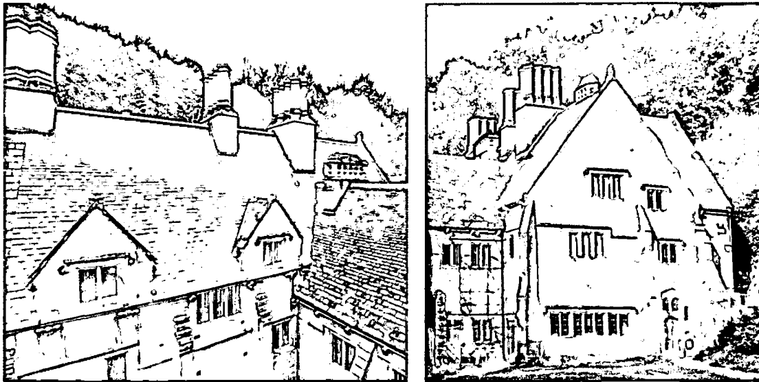
The North Range, with new roof and chimneys: Left – Across the courtyard Right – From the east
