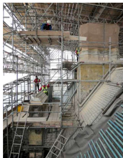
Repairs in progress
