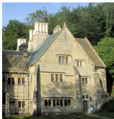
The new N range and ironing room roofs from the east
