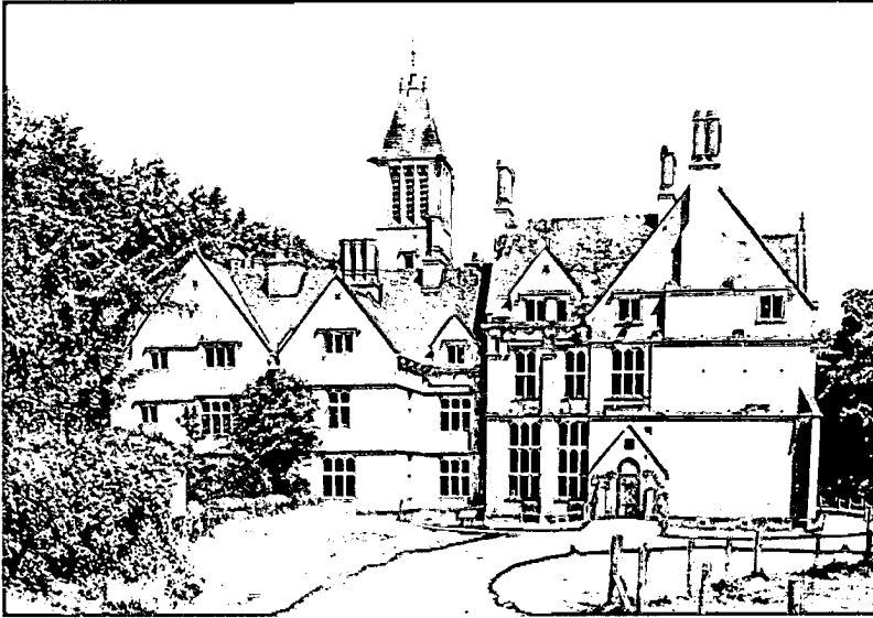
West Range of the Mansion, with new front door.
