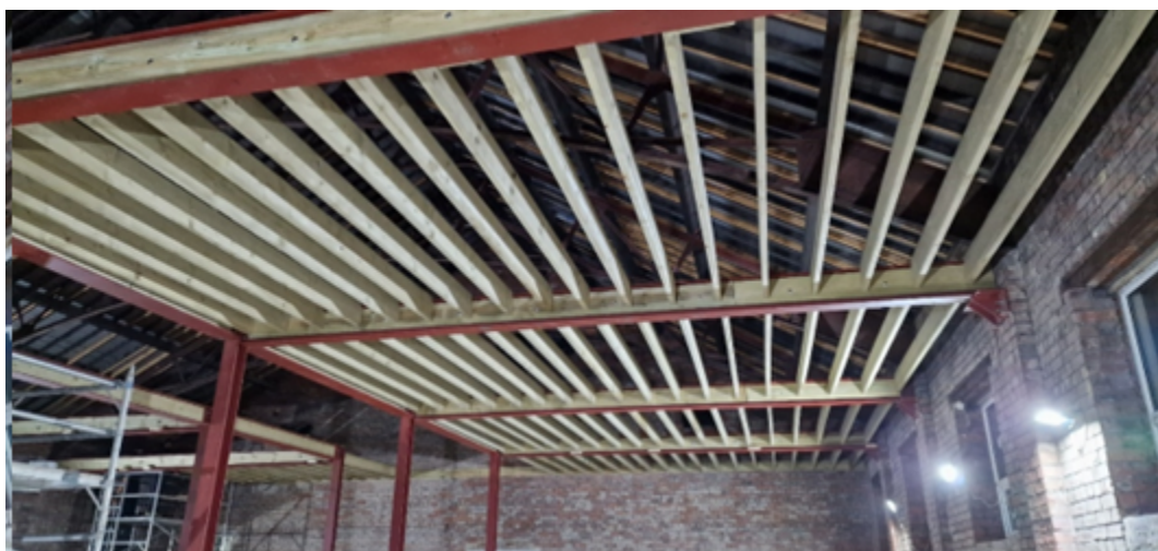
Steels installed and floor construction started.
