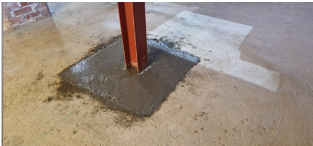
Basement footings dug out and steels installed.
