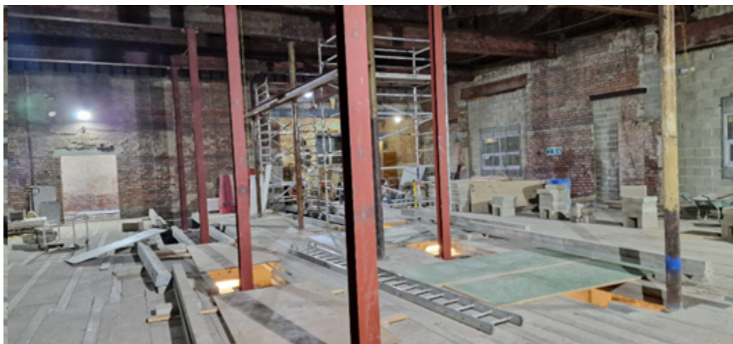
Basement footings dug out and steels installed.
