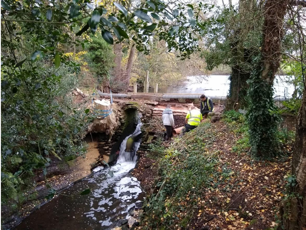
Pool spillway at start of repair work
