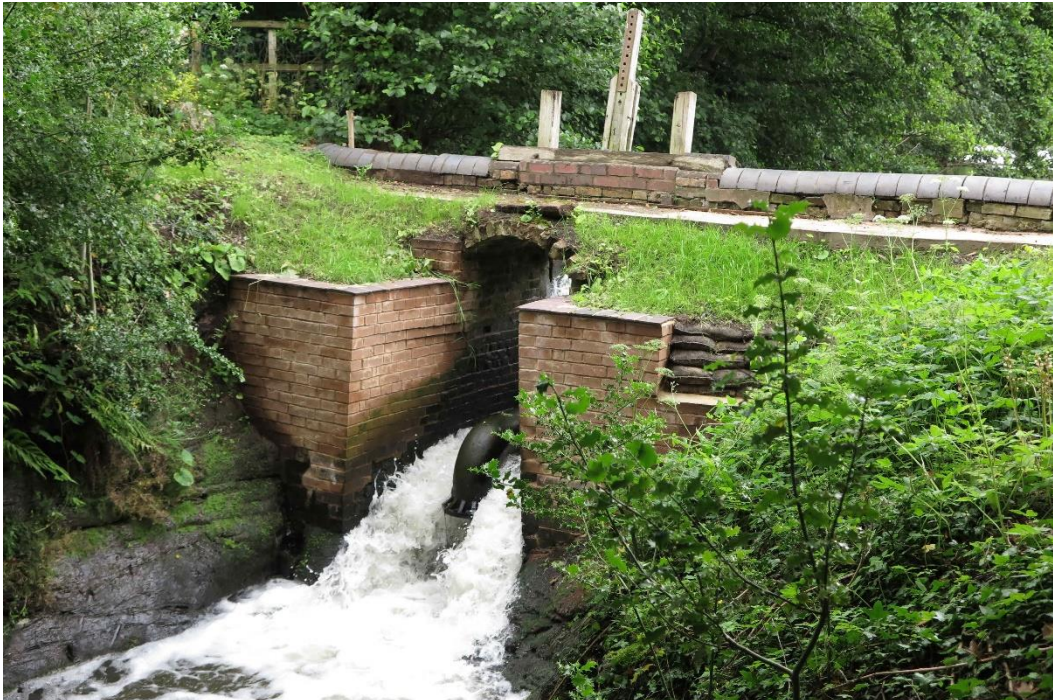
Pool spillway once repair work completed.
