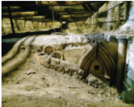
East tower base north side
