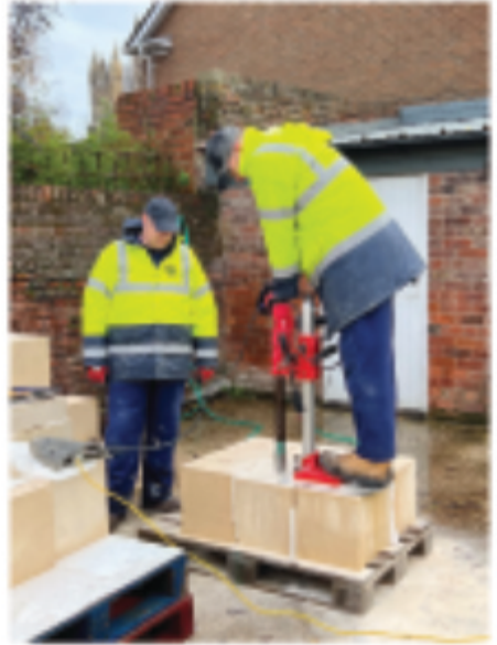
New pinnacle going up summer 2023 & Rob cutting cores into pinnacle stones with Dennis supervising
