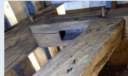
Fig 7 Carpenter's mark and reused timber
