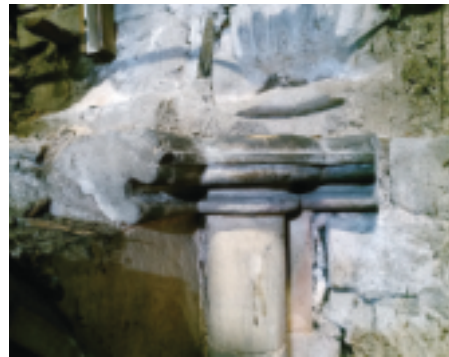
Purbeck marble moulding on ruined west side of eastern crossing north side
