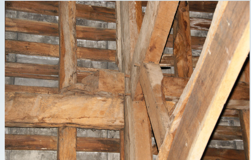
Fig 11 Medieval rafter reused as a purlin in the 1718 - 1721 reconstruction
