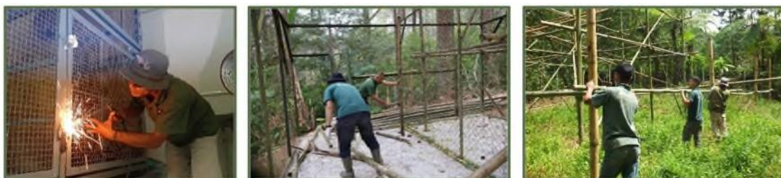
Maintenance of Animal Rehabilitation Facilities at PRS-PJ, West Java.
