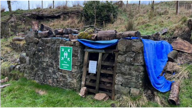
The pigsty before the refurbishment
