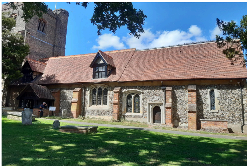
completed roof works .
