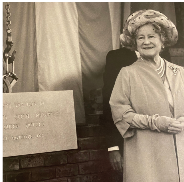
HRH The Queen Mother laying our original foundation stone in 1982
