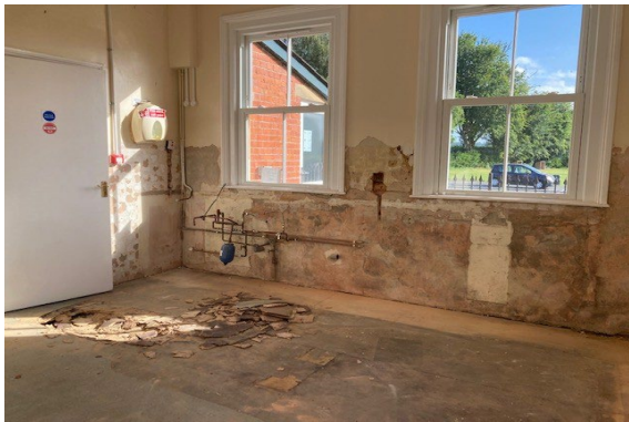
The stripped-out kitchen during its refit
