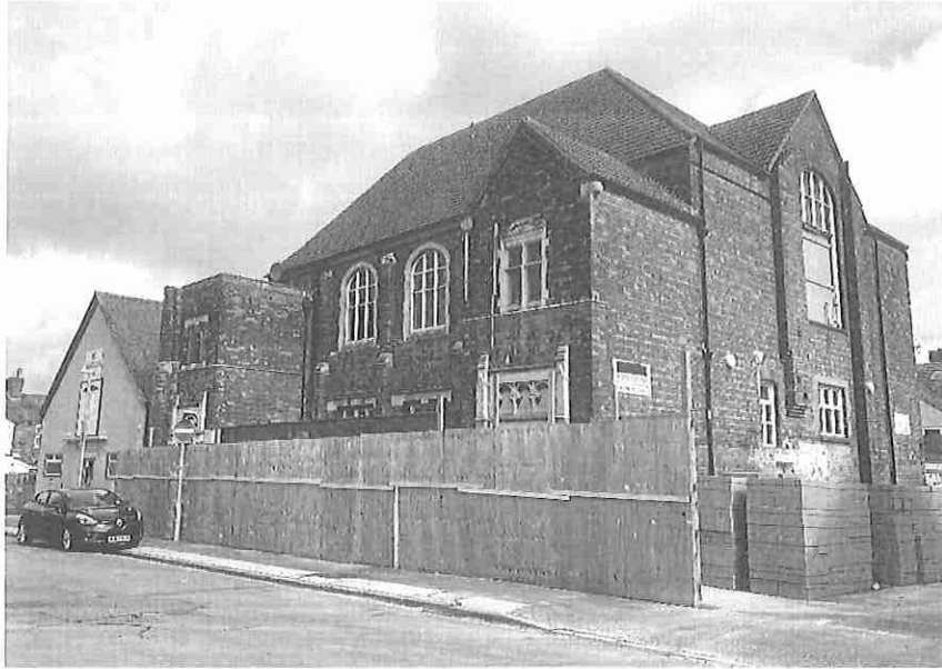
Maxwell Street School, Swindon undergoing transformation. A record of the building as it was will be preserved in the Wiltshire Buildings Record archive for future generations
