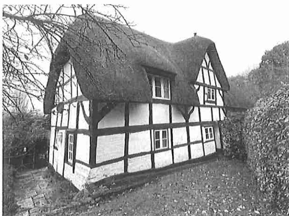
Vale Cottage, Stert. Wiltshire Buildings Record looked at this late-16 th century timber-framed building last November. It is distinguished by ogee bracing found in Wiltshire at this period.
