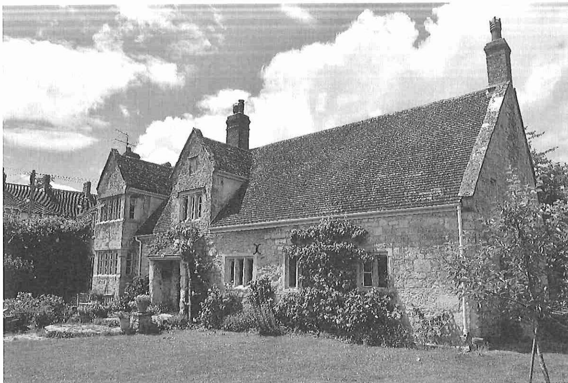
Overhouse, Tisbury. Part of phase 4 of the Dendro Project - hall ceiling dendro felling date 1532-57, hall chamber ceiling above 1575-85
