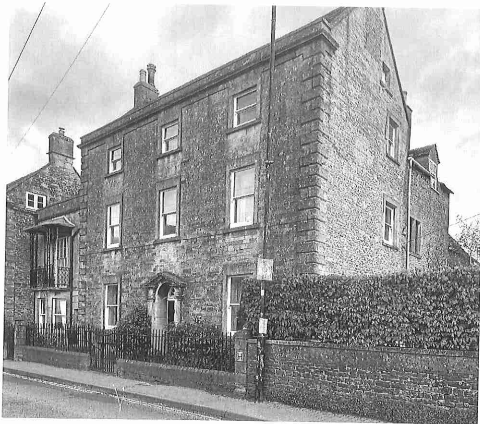
Avon House, Abbey Row, Malmesbury. This fine late Georgian house is dated 1798 and listed grade II*. It was investigated by the WBR recording team who found that it was built on top of an earlier cellar belonging to the previous house which reused early 16 th century timbers. Photo by Paul Jack
