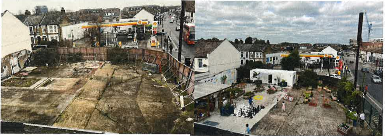
Before and after views of the once derelict site, with new developments continuing
