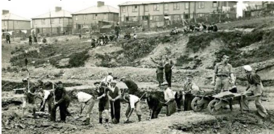
IVS volunteers in Brynmawr in 1931 constructing a swimming pool
