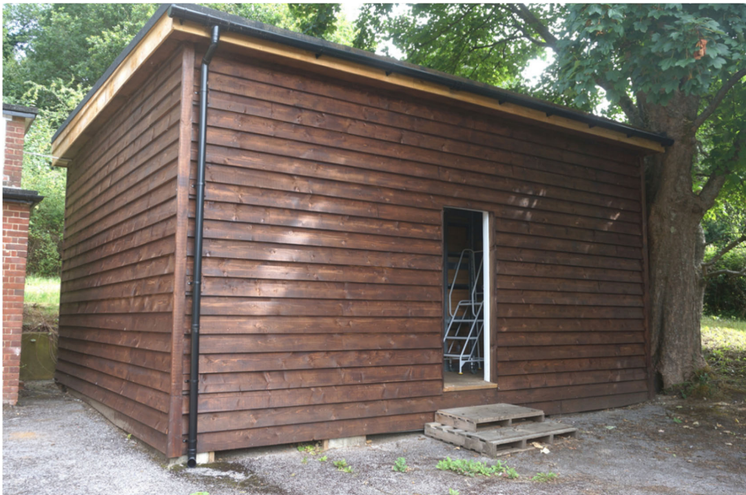
Exterior of the new Artifact store (photograph by E Corke)
