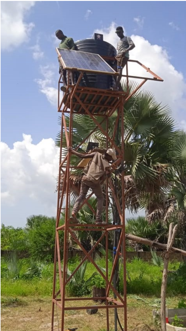
Installation of Solar Panels for the new Community Garden Borehole
