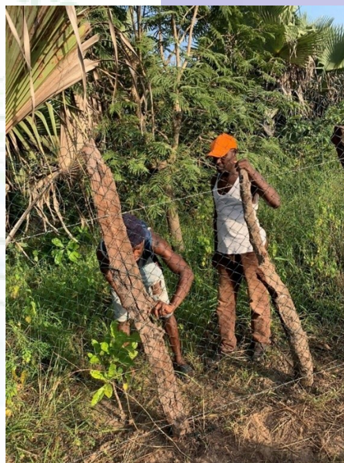
Installing fencing at the Community Garden
