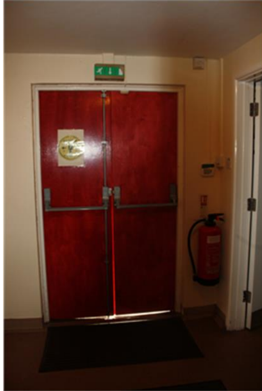
Front door – not very secure and no cover to prevent rain damage
