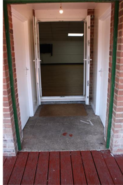
Doors from balcony do not allow level access into the Main Hall
