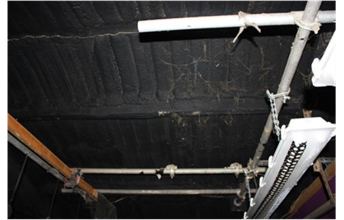
Ceiling above the stage
