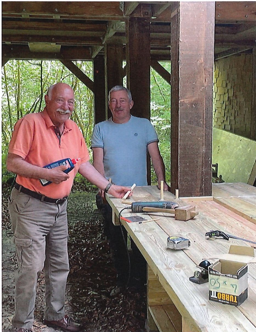
Volunteers making a new work bench in Hartford Wood
