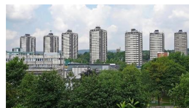
Seven Sisters tower blocks in Rochdale, Helen Cammock
