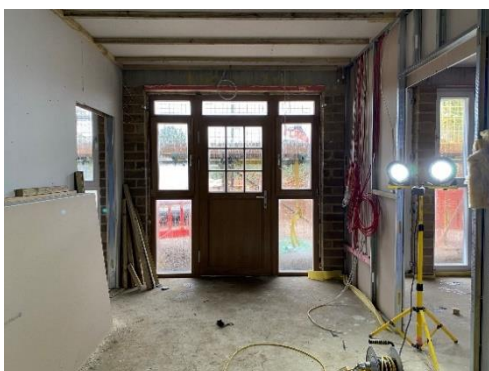
The new reception area awaiting completion
