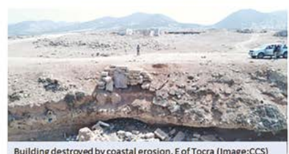
Building destroyed by coastal erosion, E of Tocra (Image: CCS)
