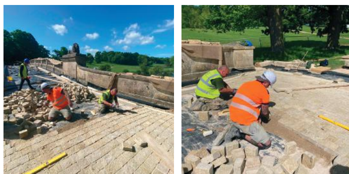
Images above: Contractors laying new stone setts during restoration.
