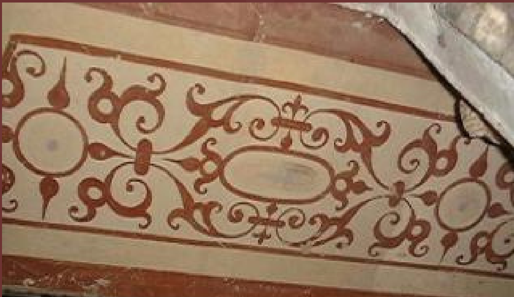
Upper lintel of window embrasure
