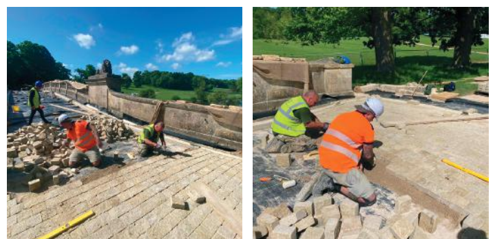
Images above: Contractors laying new stone setts during restoration.
