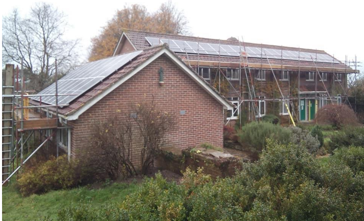
New solar panels being installed at Hilfield Friary.
