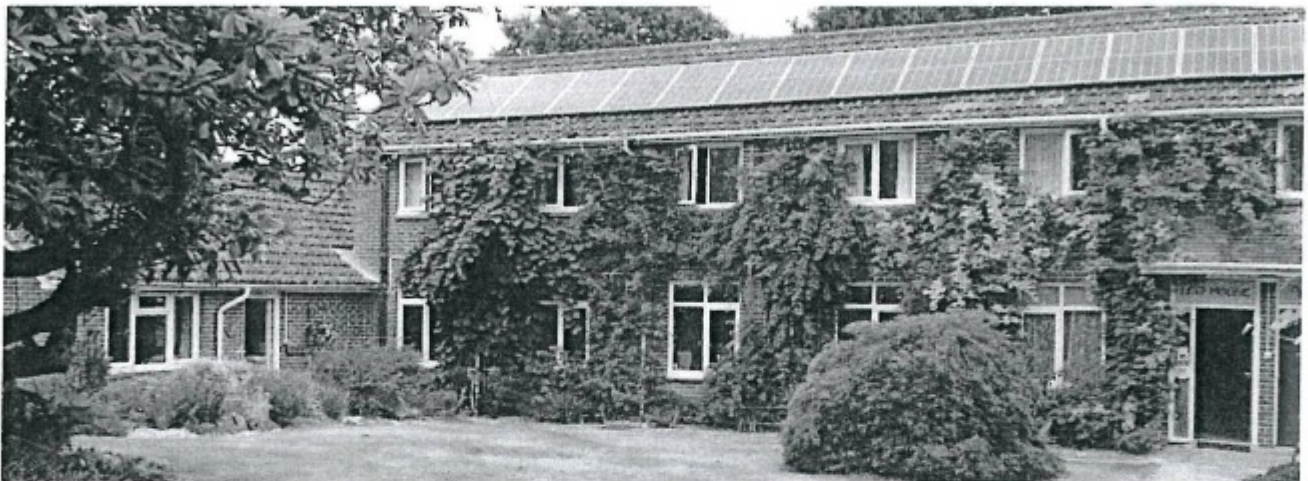
Solar panels on Leo Guest House roof at Hilfield
