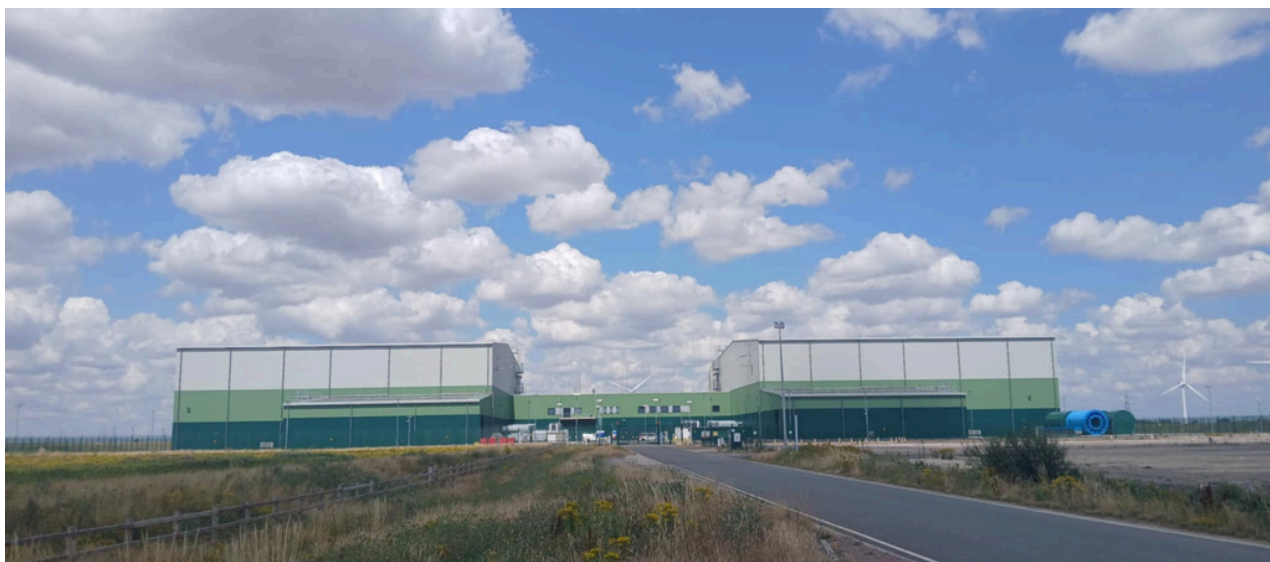
A view of Viking Link converter station in Lincolnshire
