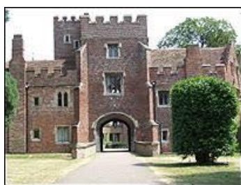
The Tower, Buckden Towers
