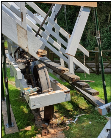
Left: the major area of rot in the left hand ladder string Right: one of the decayed sections cut off and removed
