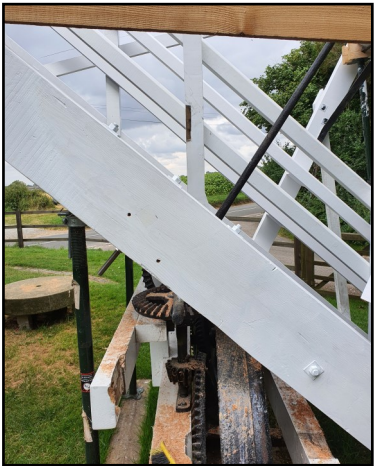
Left: the joint between the replacement section and the original string, before painting Right: after painting Photographs by Bill Griffiths, Millwright
