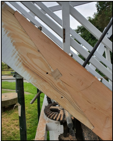
Left: the joint between the replacement section and the original string, before painting Right: after painting Photographs by Bill Griffiths, Millwright
