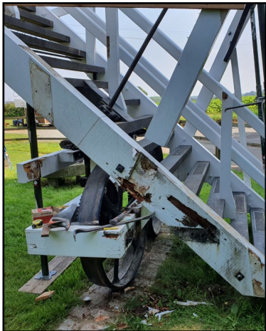
Left: the major area of rot in the left hand ladder string Right: one of the decayed sections cut off and removed
