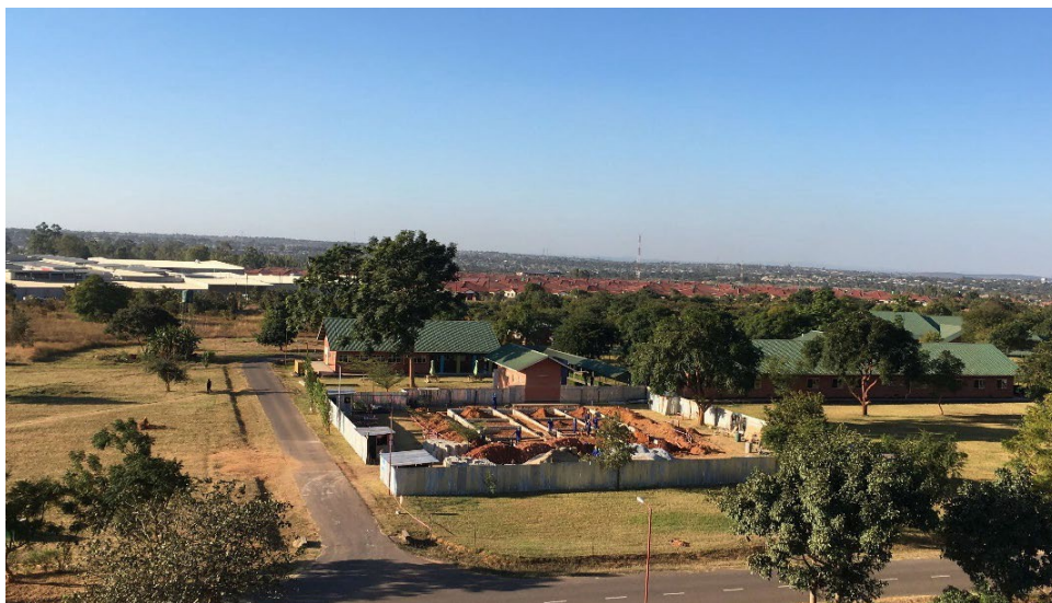
BeitCURE Hospital Lusaka. The new hostel funded by The Beit Trust
