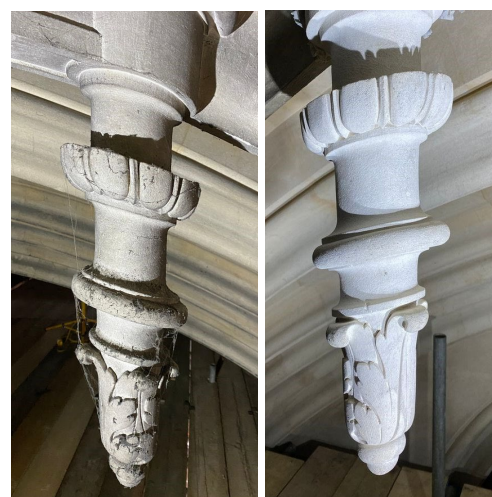
The apse corona – before and after conservation and cleaning
