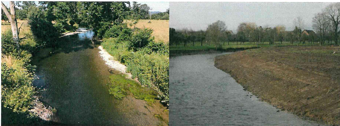
River Lugg, before and after the works
