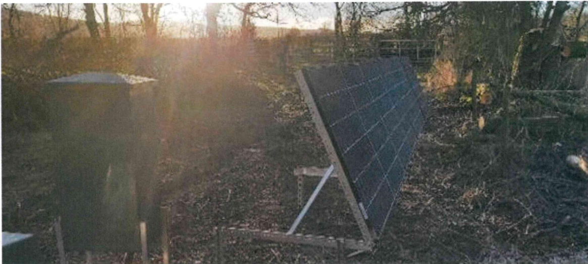
We installed a borehole and solar powered pump to provide water for cattle at Parky Meadow.
