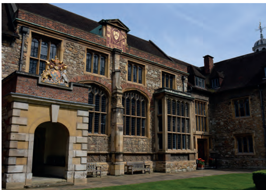
Our historic estate in central London is a major asset although the care of our Grade I and II listed buildings presents significant challenges.
