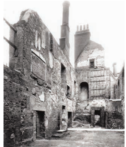
The Charterhouse suffered extensive damage in 1941 as a result of Second World War incendiary bombing. The 1950s restoration removed many 19th and early 20th century additions.
