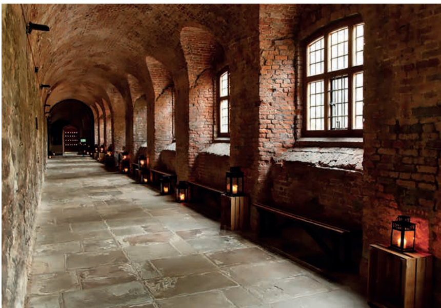
Highly atmospheric, the Norfolk Cloister encompasses numerous issues that affect the Charterhouse's historic fabric – uneven floors, a lack of adequate heating, and poor thermal control from single glazing.
