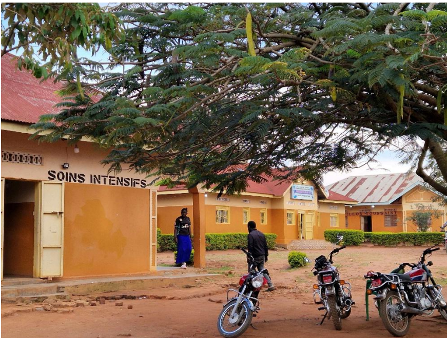
New intensive care block, Aru Cité Hospital
