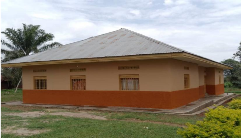
Renovation of maternity and Ekanga health centre, Aru coordination.
