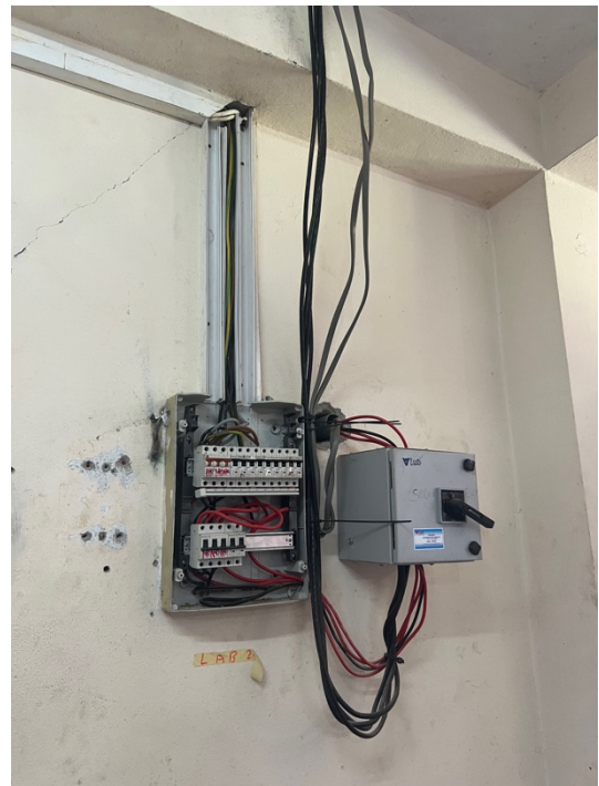
Unsafe fuse box with wires
