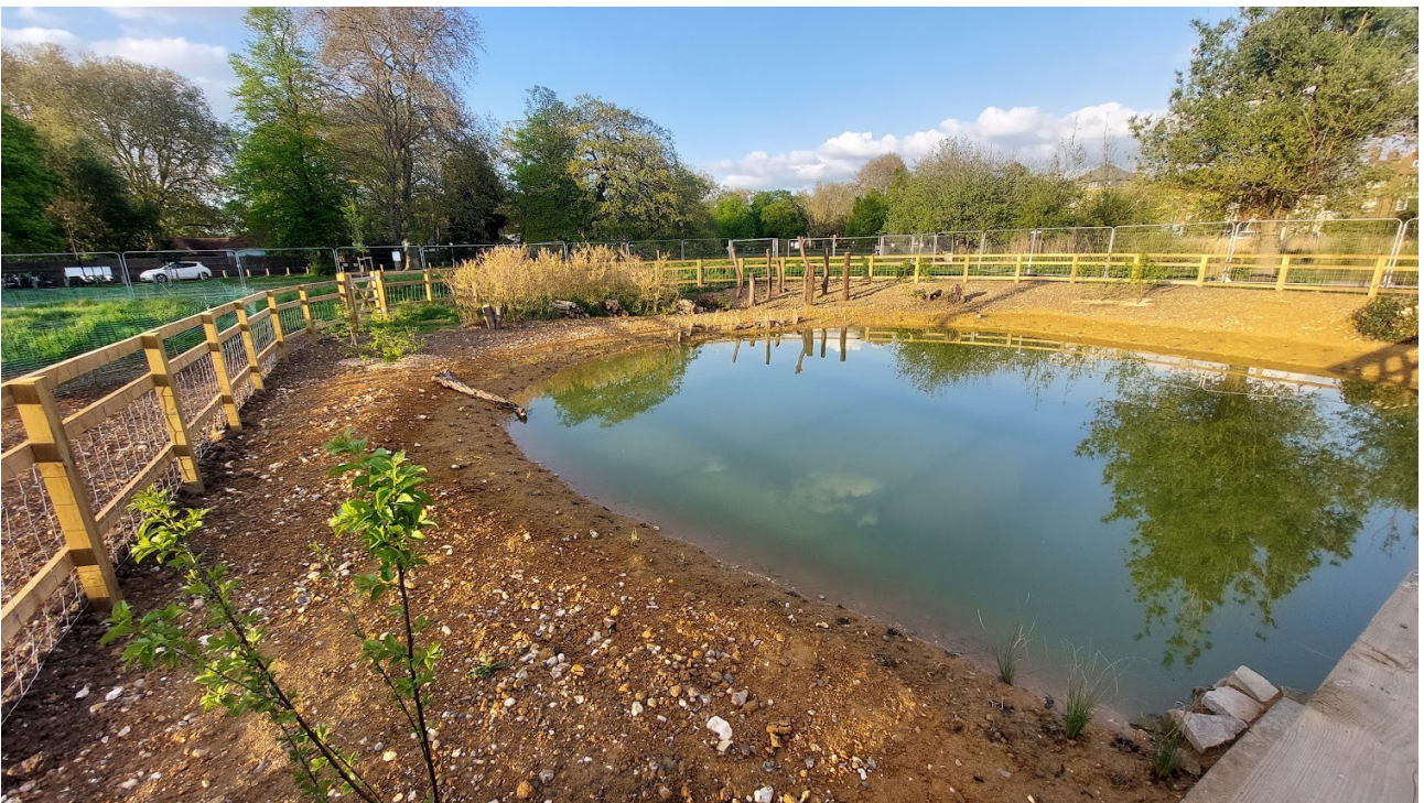
Wetland project during construction, April 2025
