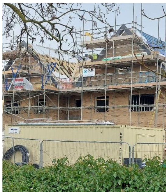
Ebenezer Lodge, Swavesey under construction
