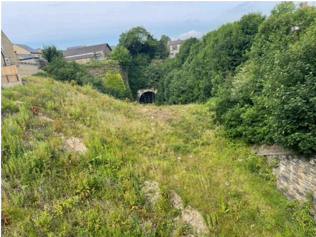
Closed: Greenside Tunnel. Photo: John Baron
