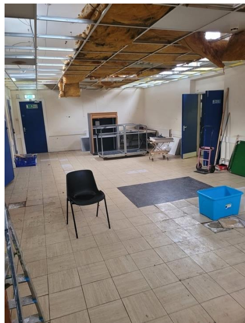
OCC - Much work to do!
