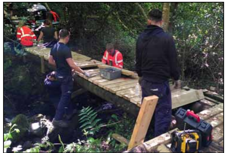
Bridge restoration by WPD apprentices - June 2022
