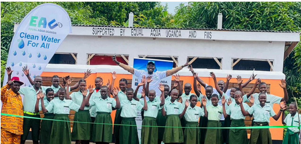
Sustainable Pit Latrine at Ebenezer Primary School, Eastern Uganda
