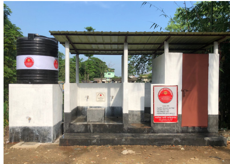
Public toilet under construction at Lala Bazaar
