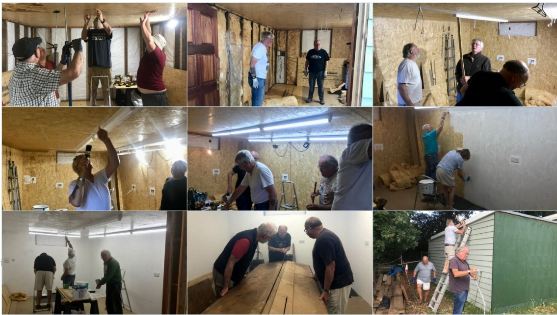
Finishing room (May – July 2023)
