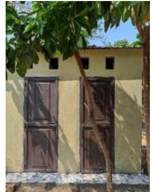
Completed toilet with doors
