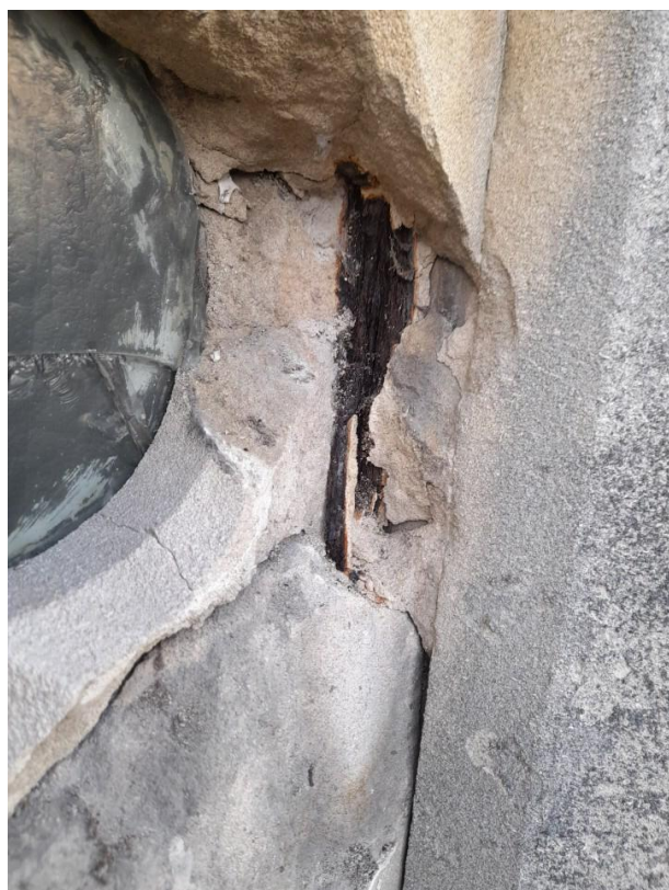
Figure 2 Damaged stonework requiring urgent attention.
