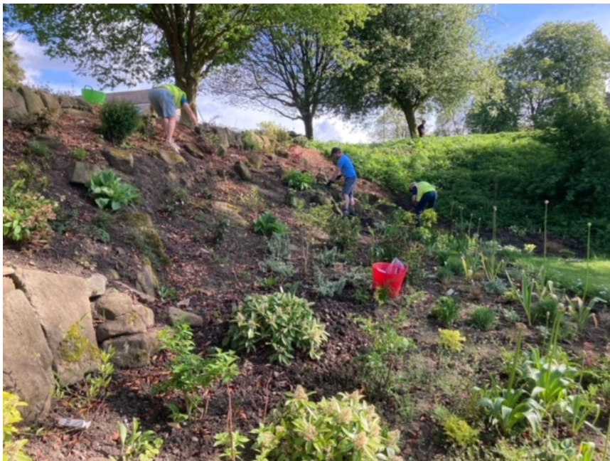
New Planting Embankment Riverside Gardens 2022
